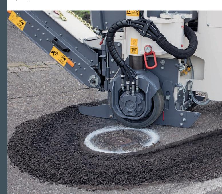
1 - 2 | The electronically controlled travel drive makes high-precision milling possible - such as around road installations, for example.
