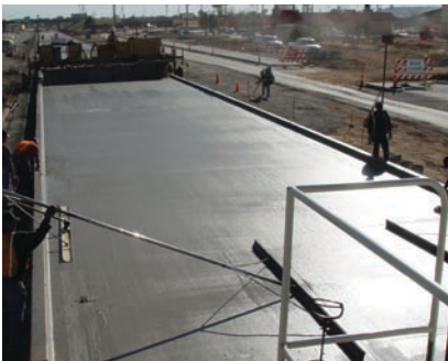
Excellent visibility of slab behind paver.
