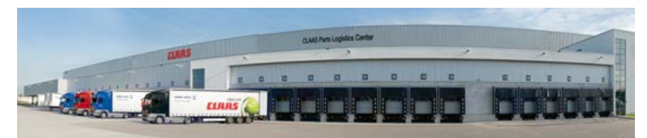
The CLAAS Parts Logistics Center in Hamm, Germany, stocks more than 155,000 different parts and has a warehouse area of over 100,000 m 2 .
